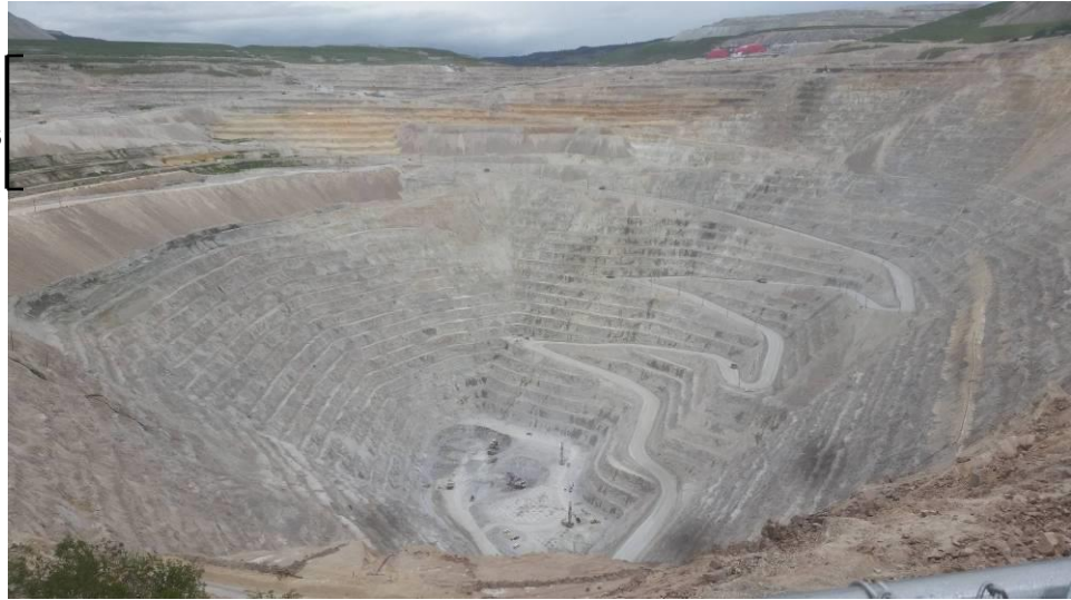
Figure 2 View of the Valley pit at the Highland Valley Copper Mine, viewed towards the southeast. The thick layer of unconsolidated sediments is shown.
